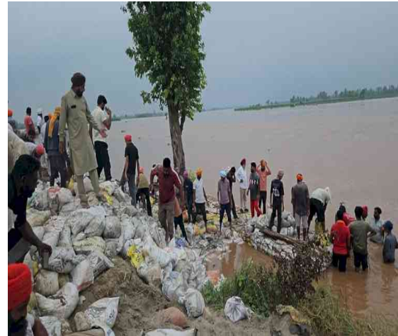
Villagers strengtheing the embarkment of river in Ferozepur
